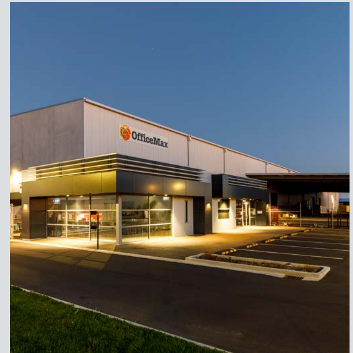
Christchurch distribution center
